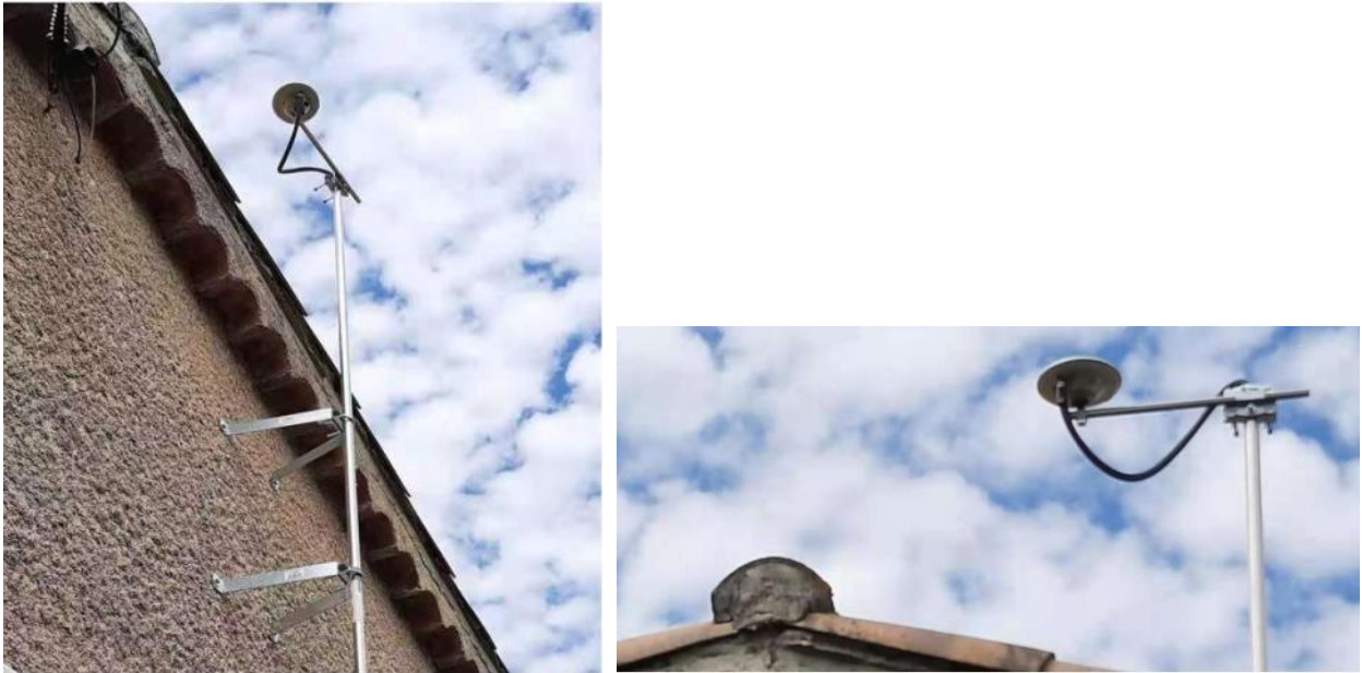
Figure 6: Base Station Antenna Installation
